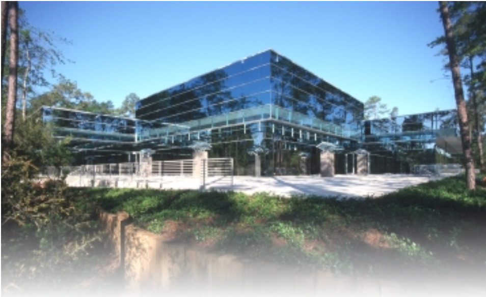
THE VENTURE TECH BUILDINGS in The Woodlands house biotechnology and other research firms.
