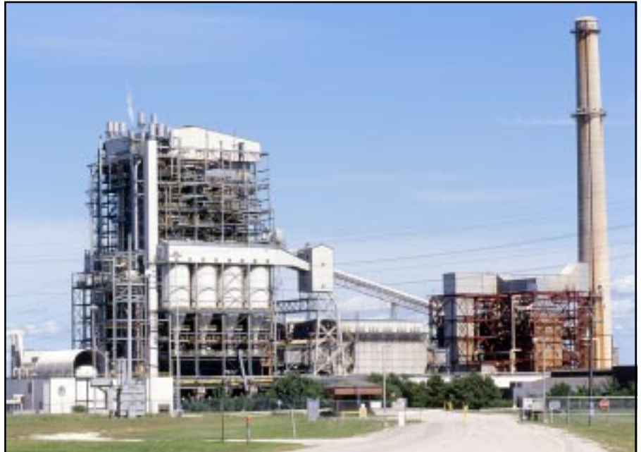
THE CHOICES CONSUMERS HAVE NEXT JANUARY will depend on whether their power is currently provided by a municipal electric utility, an electric co-op or an investor-owned utility.
