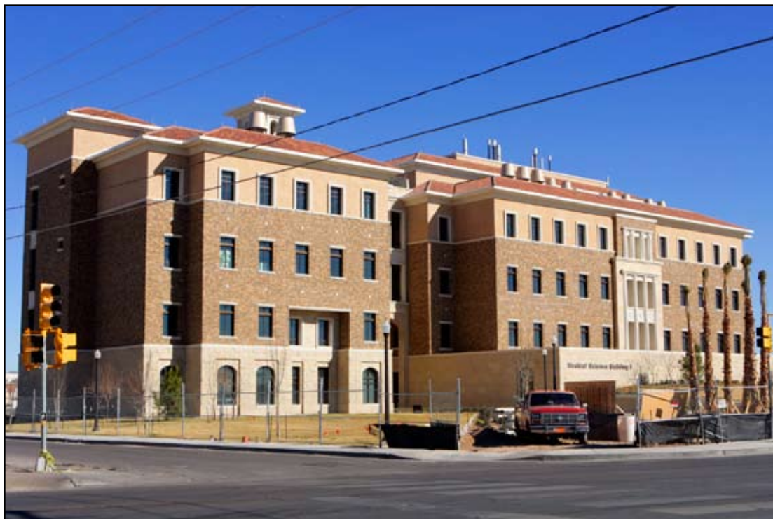
THE TEXAS TECH UNIVERSITY Health Sciences Center School of Medicine El Paso has completed the first of two buildings that will support the expansion of its two-year program to a full four-year program.
