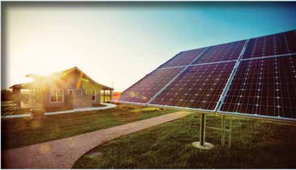
Bluebonnet Electric Cooperative's energy-efficient demo home in Brenham.
