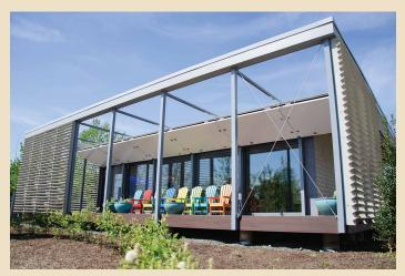
Thin, flexible, marine-grade, plastic, solar photovoltaic panels are extremely lightweight, allowing a homeowner to easily raise and lower the shutters manually. The panels have much greater impact resistance than glass to prevent damage when struck by debris.
