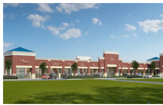
RIVERSTONE SHOPPING CENTER New Retail Center for Lease NEC Riverstone & Crosslakes, Missouri City, TX
