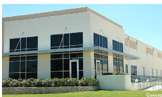
GILLINGHAM DISTRIBUTION CENTER Up to 76,050-SF Build to Suit on 5.6 Acres 1601 Gillingham Ln, Sugar Land, TX
