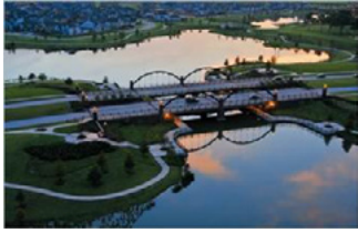
TELFAIR/HWY 59 COMMERCIAL TRACTS +/- 187 Acres for Commercial Development Hwy 59 & University Blvd, Sugar Land, TX
