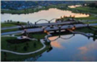
TELFAIR/HWY 59 COMMERCIAL TRACTS +/- 187 Acres for Commercial Development Hwy 59 & University Blvd, Sugar Land, TX
