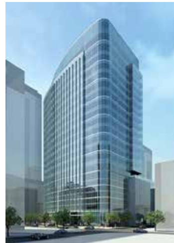
1110 Main Partners: An investment partnership with a connection to Hilcorp Ventures is under construction on an office building on the site which used to house Macy's.
