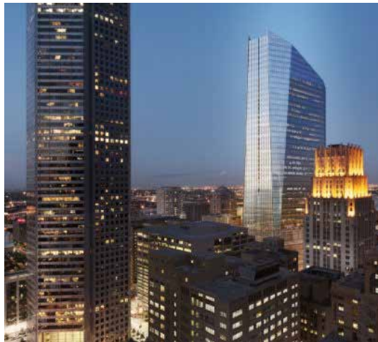
609 Main: Houston-based Hines has started work on a downtown block at 609 Main where it will build a 1 million square foot, 47-story tower.
