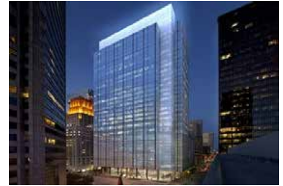
Capitol Tower: Skanska USA Commercial Development is making plans to demolish the former Houston Club building where it has plans to build a 755,000 SF tower at the site.
